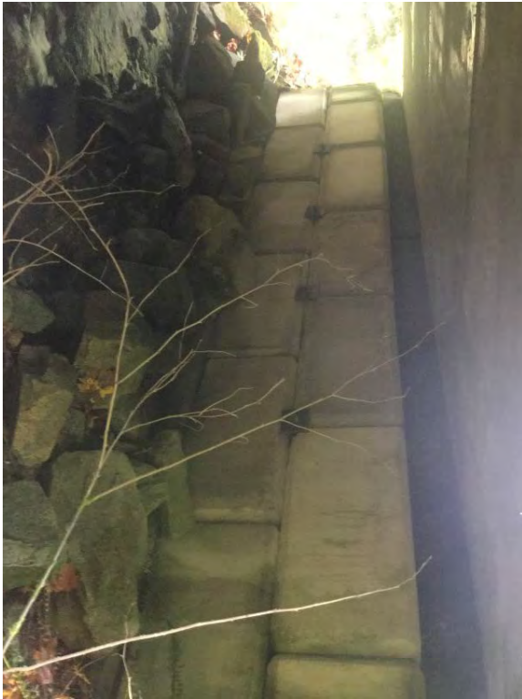
Right Bank Abutment when facing downstream
